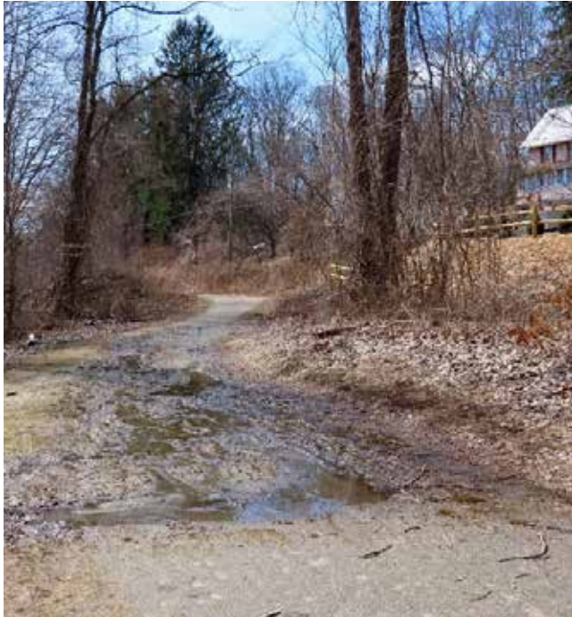
ALSPT Trail surface erosion from rain event
