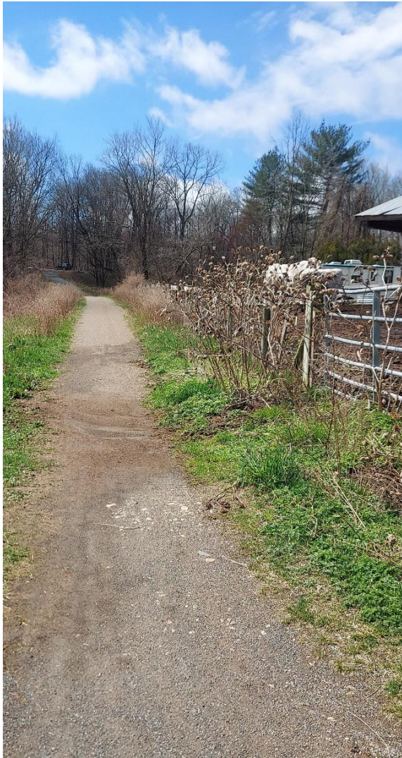
Figure 12 Manure contaminated stormwater flows across the Airline Trail from an adjacent farm.
