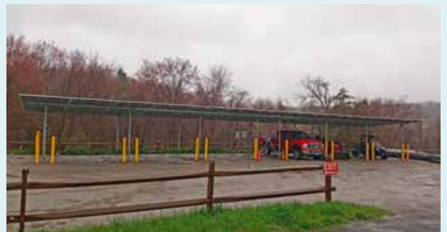
Aquila's Nest Vineyards installed a 35.1 kW carport solar PV system at their farm located in Newtown, CT in 2024.
